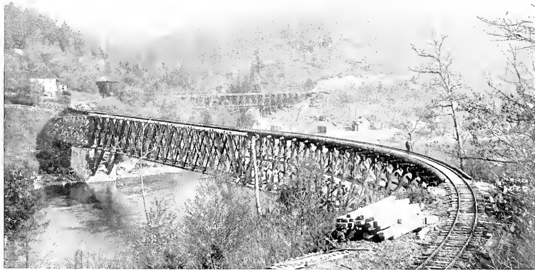
OLD B. & O. RAILROAD BRIDGE OVER THE CLARION RIVER
