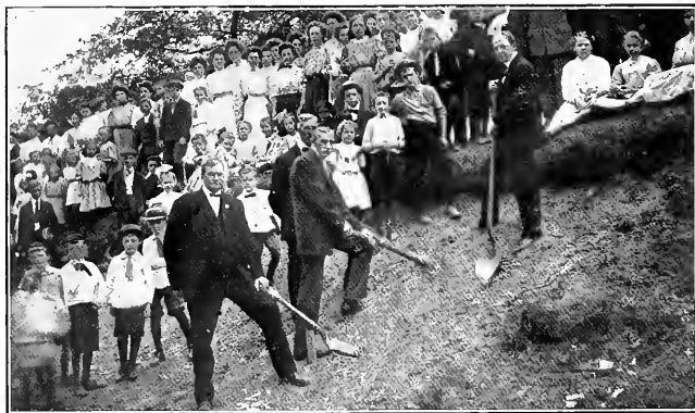
BREAKING GROUND FOR THE NEW DORMITORY.
