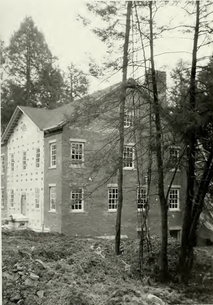
The side view of the house shows how large the three and a half story house looks like on the outside.
