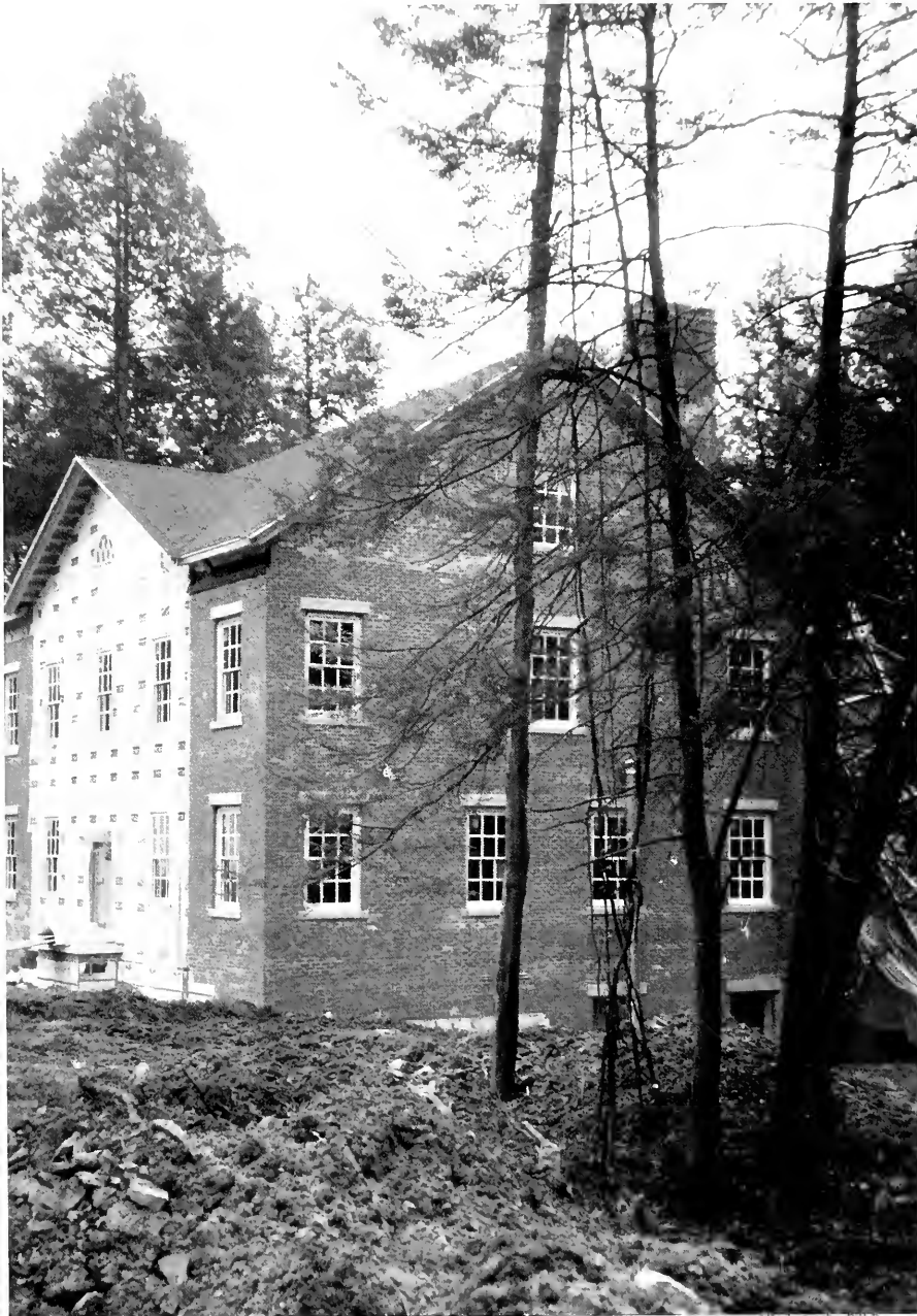
The side view of the house shows how large the three and a half story house looks like on the outside.
