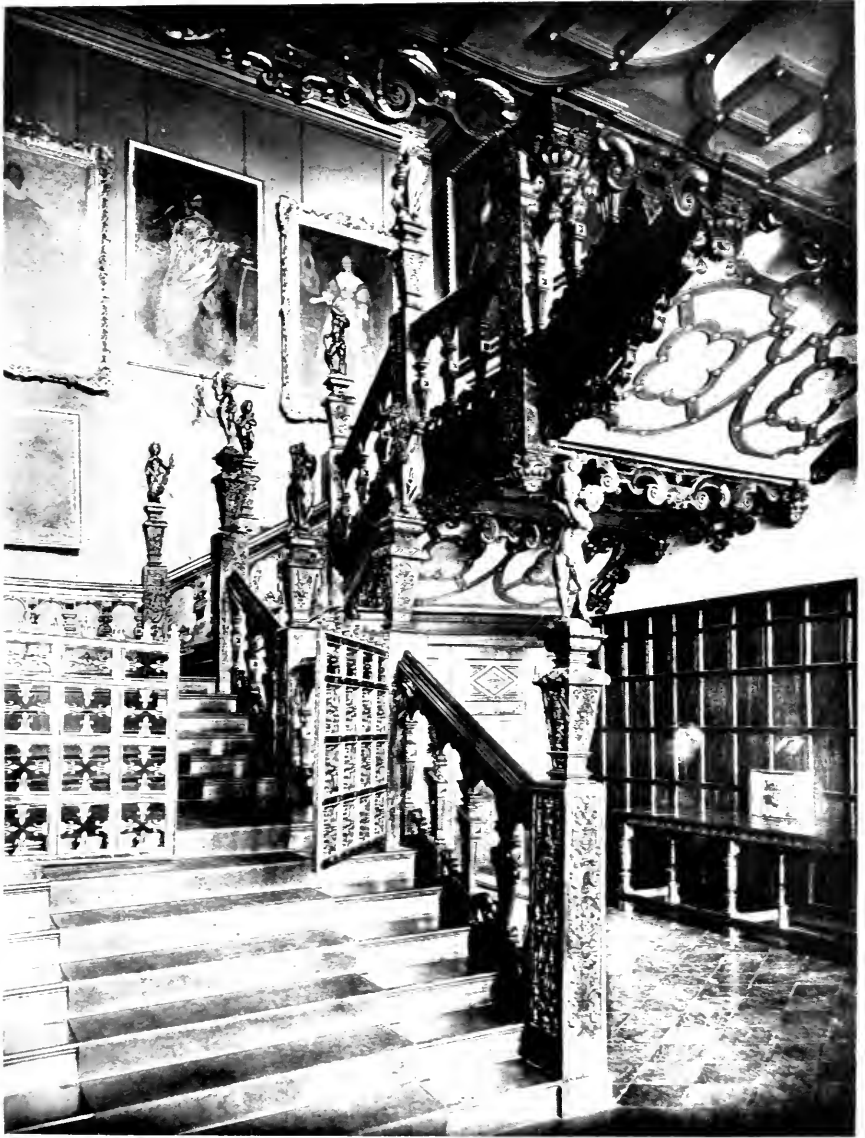
Fig 11 STAIRCASE AT HATFIELD HOUSE
