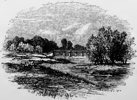
The Foot-Bridge at the Mill.
