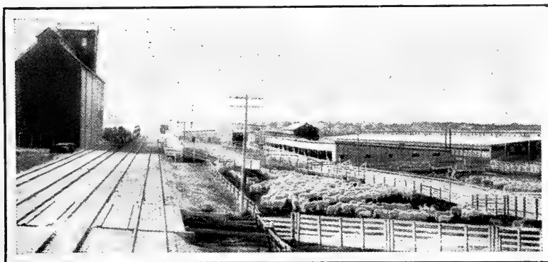
AN ILLINOIS FEEDING AND SHIPPING YARD.
