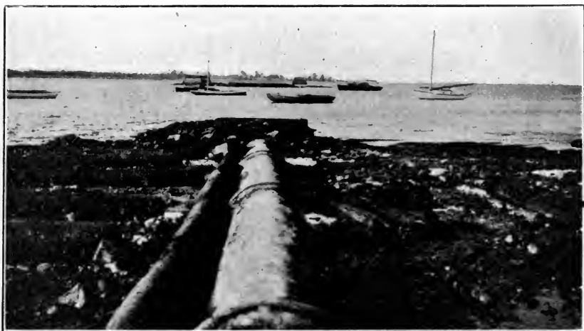
FIG. 1.—One of three main sewers emptying untreated sewage into the mouth of a river. This sewage combines with that from several other large cities and flows over extensive shellfish grounds.
