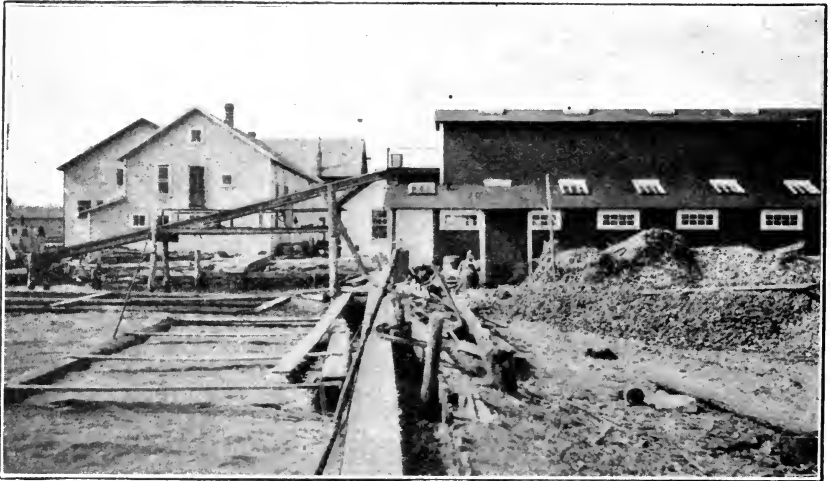
FIG. 6.—Oyster floats located near a shucking establishment. The small building in the foreground is a privy used by 100 to 150 men. The drainage from this vault seeps through the loose soil and wooden wall into the water which bathes the floats. Drainage from decaying shell heaps and the washings from these oysterhouses likewise flow into this same water. Analysis of this water and oysters on the floats showed contamination.
