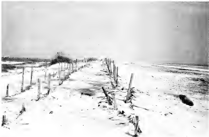
Figure 6-33. Sand Fence Deterioration Due to Exposure and Storms
