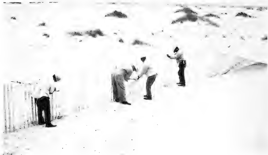
Figure 6-29. Erecting Snow-type Sand Fencing
