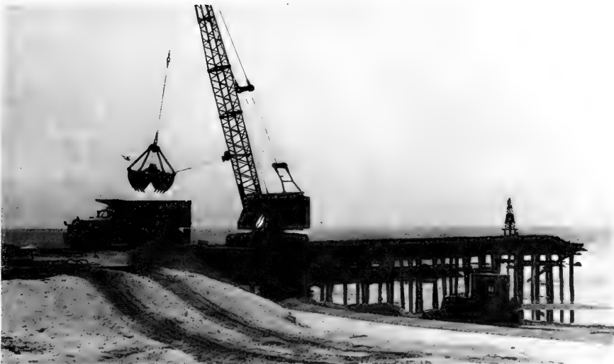
Excavating sand from the borrow area
