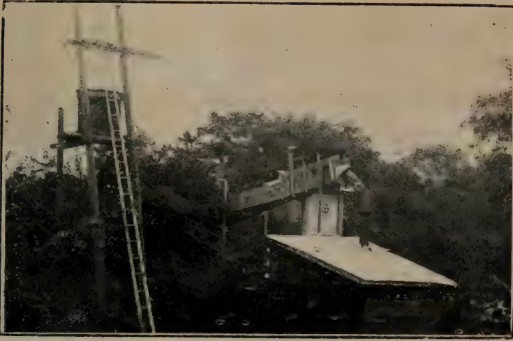
Pumping Station for Drainage at KeKung Village 科貢鄉之排水機
