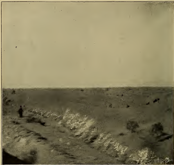
BUNDLES OF FAGOTS USED AS A SAND BARRIER TO PROTECT THE RAILWAY AGAINST THE DRIFTING SAND
