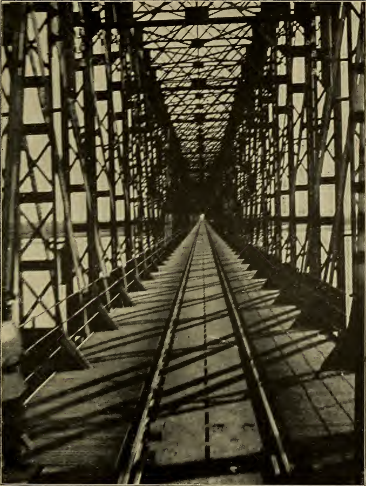
GREAT BRIDGE ACROSS THE VOLGA RIVER AT BATRAKI ON THE TRANS-SIBERIAN RAILWAY
