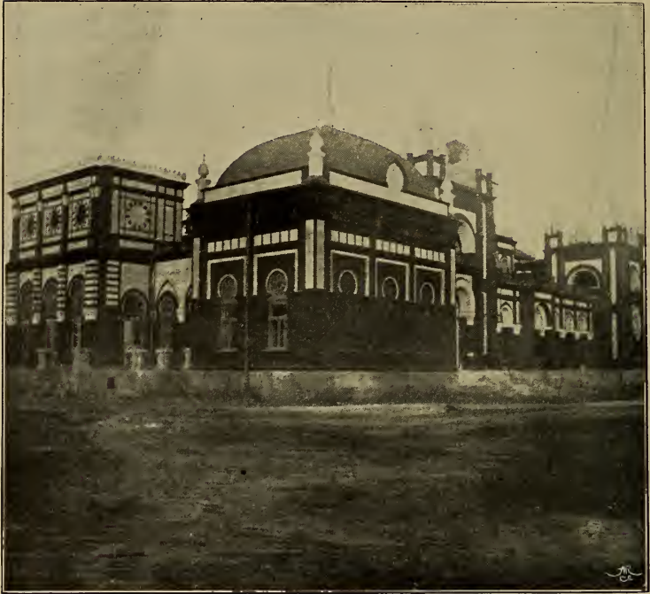
NEW PALACE BEING BUILT BY RUSSIA FOR THE AMEER OF BOKHARA, NEAR THE STATION IN THE NEW, OR RUSSIAN, TOWN OF THAT NAME
