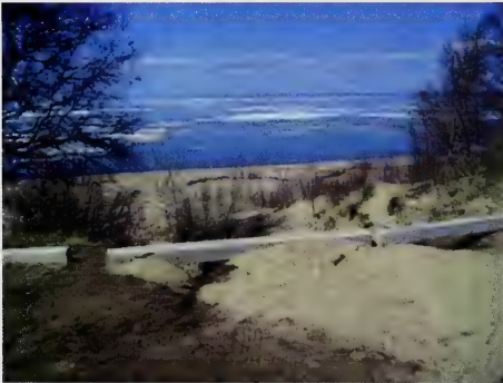
Figure 8. Erosion associated with trails from pull-offs.
