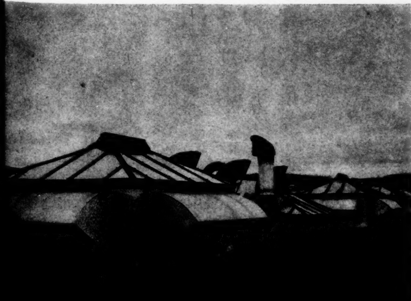
Fig. 1. How the skylights appeared when raised with filters in place of the glass on the sides.
