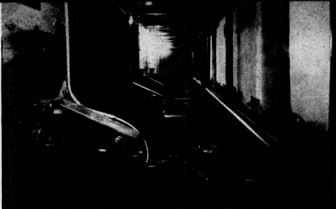
Fig. 1. Aisle behind the boilers showing the coal bin and stoker driving mechanism at the left and the rear of the boilers at the right.
