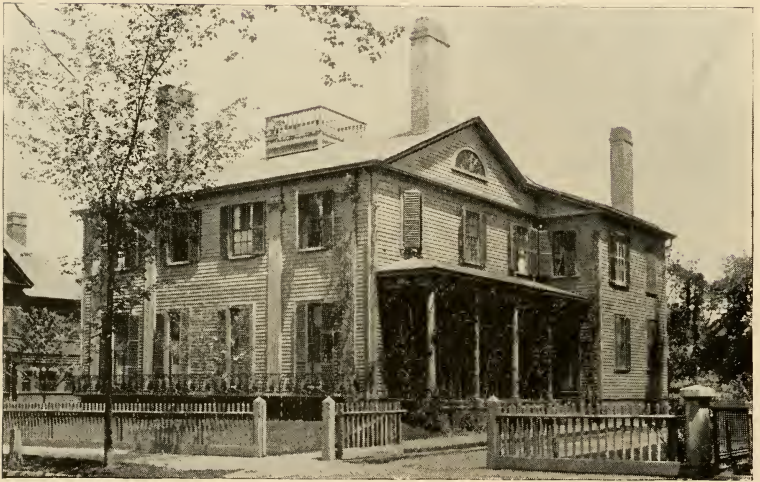
55 Chestnut street, home of George Merriam from 1848 until his death in 1880. The house was built in 1824-5 by Simon Sanborn for Edmund Dwight, and was afterwards occupied by Judge Cummings, Jonathan Dwight, 3d, and Horace Draper, who was of the firm of Draper & Bailey. The projection in the rear on the right of the building was built by Mr. Merriam.
