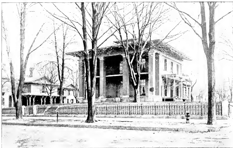
The residence of the late Hon. Chester W. Chapin, 149 Chestnut street. Erected in 1844.
