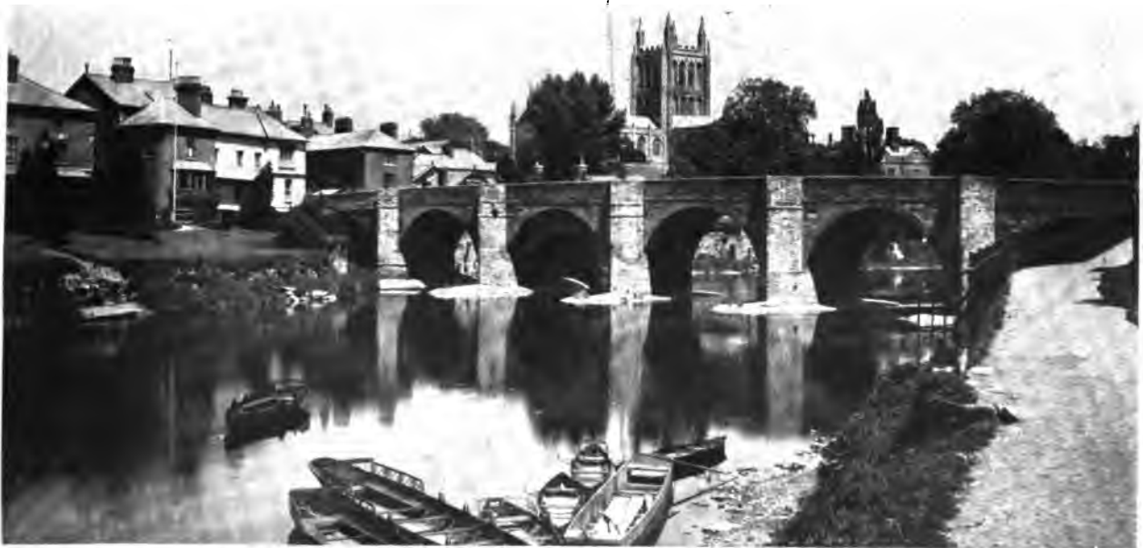
Photograph of the Wye Bridge and Cathedral. Three Sketches Drawn from this Photograph are Shown in Figure 25.
