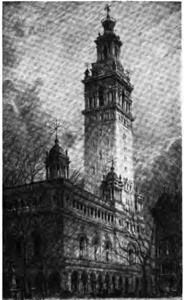
Sketch by Hugh Ferriss. Madison Square Garden, New York. McKim, Mead & White, Architects.
