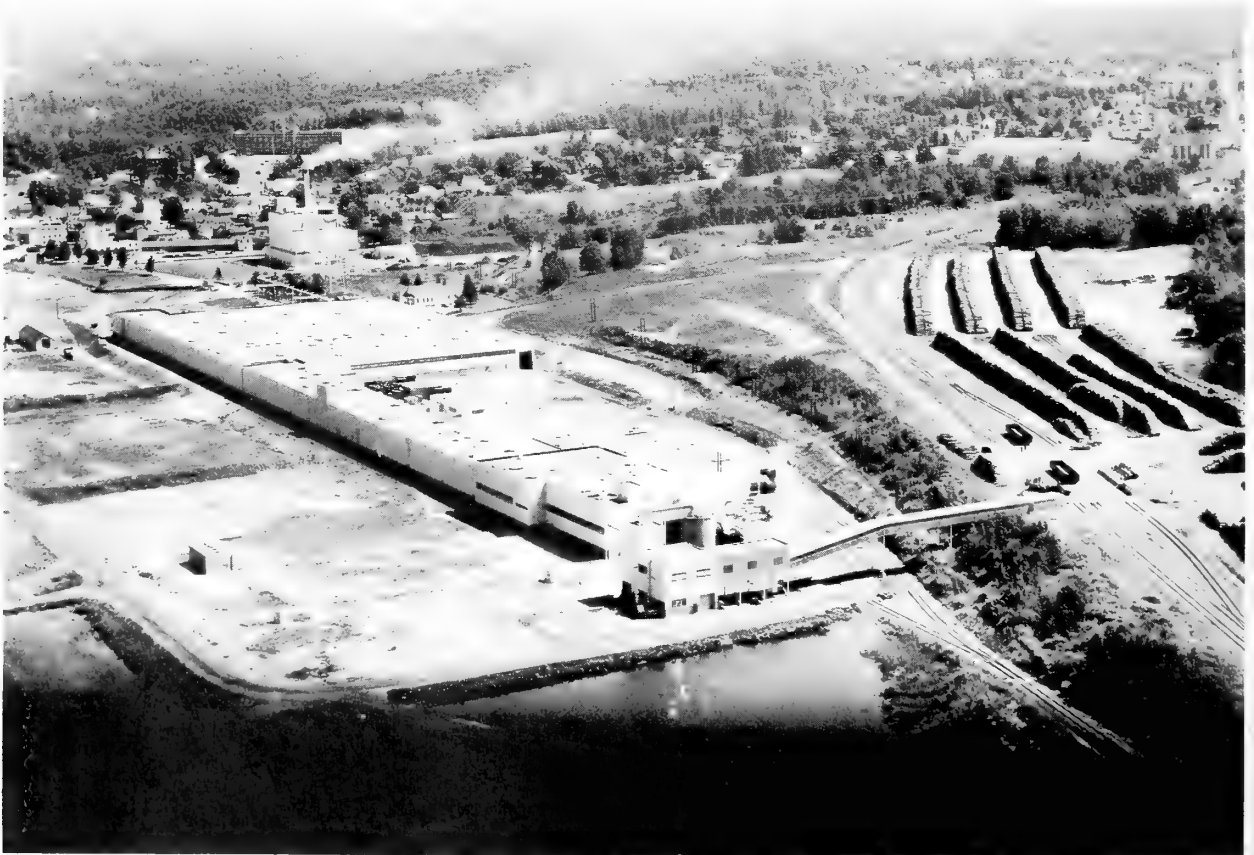
Figure 3.—This new fibreboard mill at L'Anse represents new jobs and new incomes for the Upper Peninsula. (Photo courtesy Celotex Corporation, L'Anse, Mich.)
