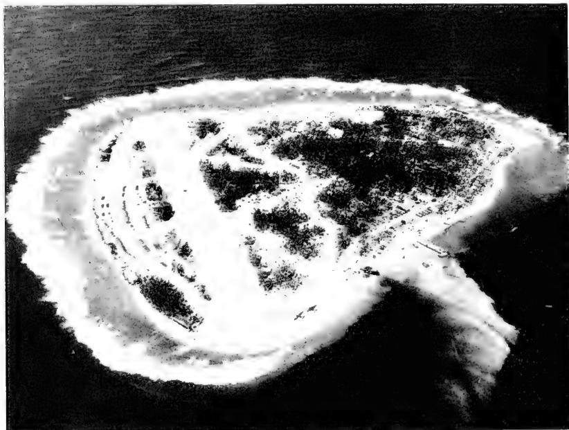
1. FALALOP ISLAND, ULITHI ATOLL. SHOWING THE AMOUNT OF CLEARING OF THE SMALL ISLAND FOR MILITARY INSTALLATIONS
