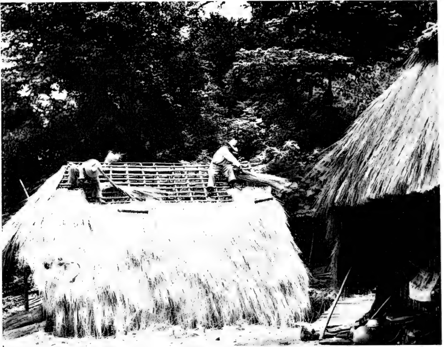
1. Construction of native dwelling (ranchito). Usually the roof must be replaced every 5 years. Neighbors often cooperate in accomplishing this task.
