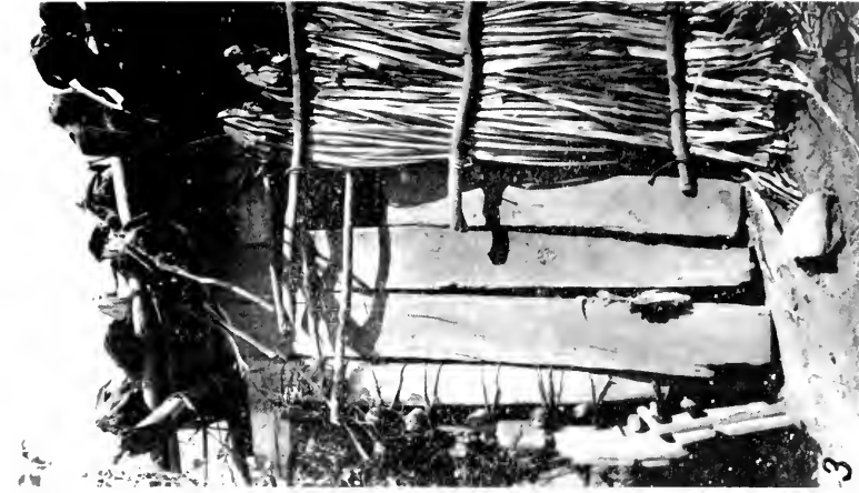
Building materials (Alepie): 1. Ratomera used in thatching a ruka. 2. Vine (voque) used in building fences and ruka. 3. Detail of a chicken coop. (Note the manner of keeping ratomera in place. All attaching is done with vines.)
