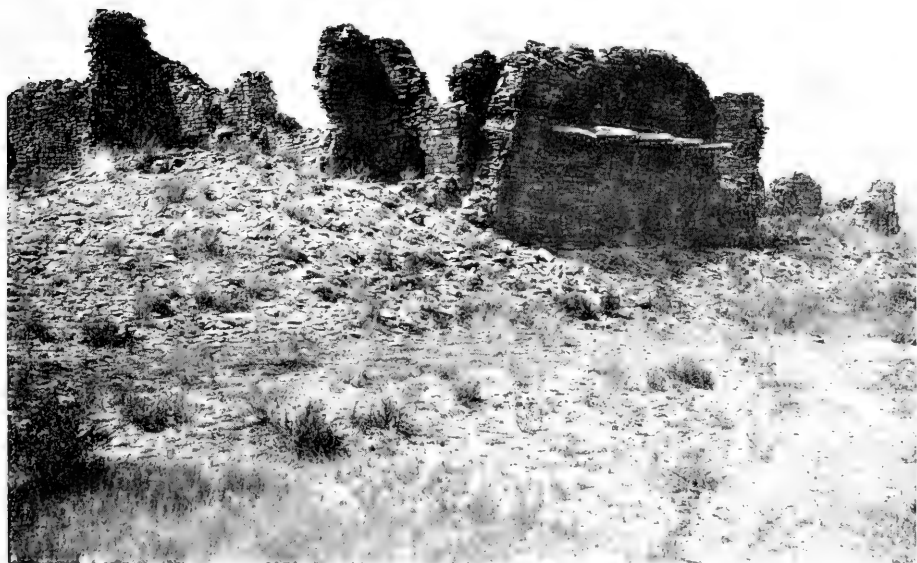
B. Northeast corner of north wing, with second-story ceiling beams projecting from outer north wall. (Photograph by Victor Mindeleff, 1887. Courtesy of Bureau of American Ethnology.)
