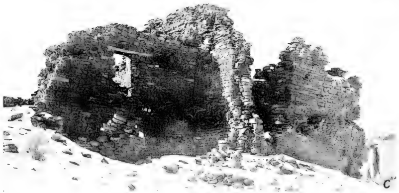
a , The outer south wall, from the southeast; b , south end of Room 45B(?); c , east tier rooms, south wing.
