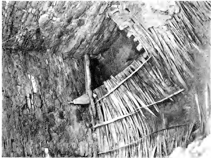
A. Hatchway in southeast corner of Room 20B. (Photograph by O. C. Havens, 1923.)
