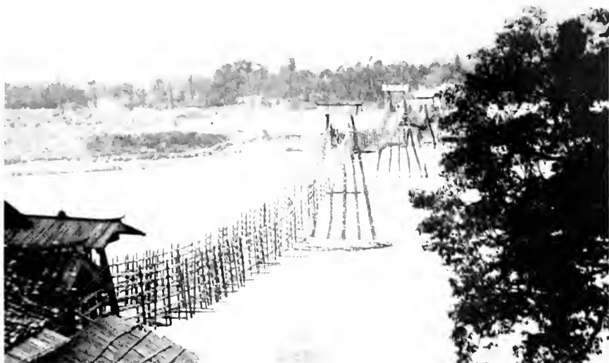
1. A typical bamboo cable or "rope" bridge at Kuanhsien. Similar bridges are found at So-ch'iao, Wen-ch'uan, Li-fan, Wei-chou, and Mou-chow in western Szechwan.
