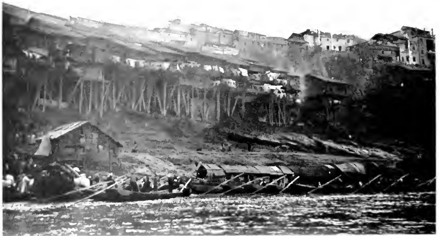
2. View of Chungking from the Yangtse River. On the shore are Chinese wooden boats; higher up, Chinese houses on high wooden posts to keep them above the river in high water; and still higher are temples and other buildings of Chungking.
