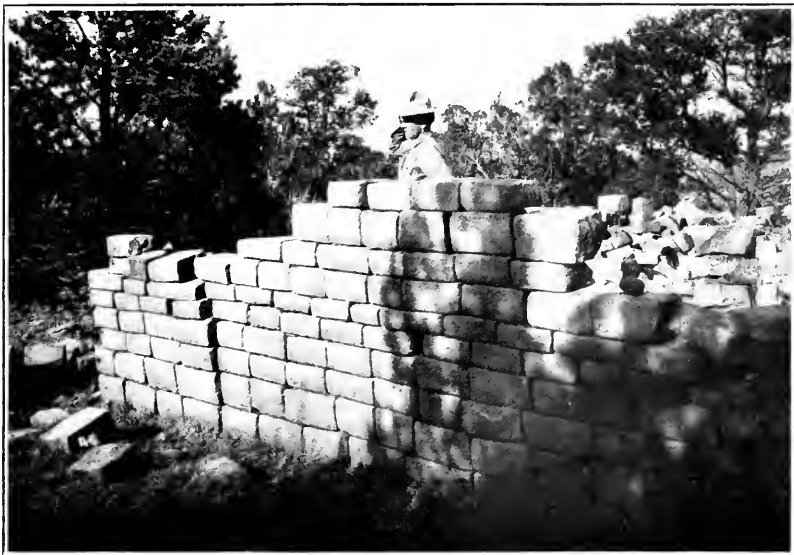
FIG. 54.—Character of masonry shown in one of the house-groups of the compound. Note the failure of the builders to “break” the joints and the consequent weakening of an otherwise excellent wall. The face of the stones is pecked to smoothness and all the stones are artificially squared. Photograph by Nusbaum.
