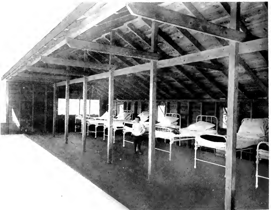
FIG. 2. LOOMIS SANATORIUM, SULLIVAN COUNTY, NEW YORK. SLEEPING GALLERY IN GUILD LEAN-TO
