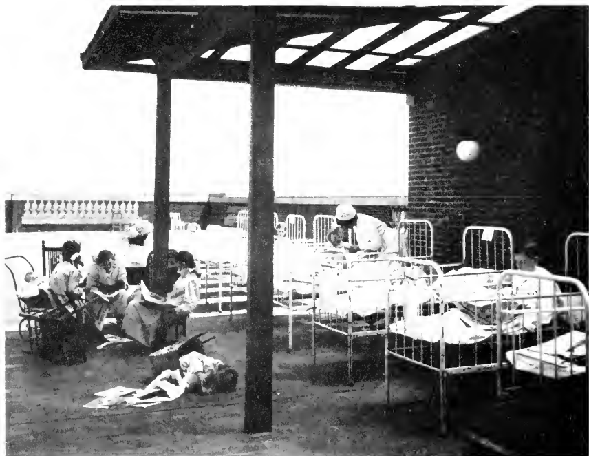
FIG. 2. BELLEVUE HOSPITAL, NEW YORK CITY. ROOF WARD FOR CHILDREN
