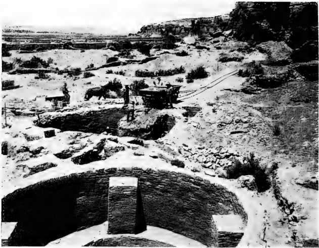
FIG. 131.—Excavating one of Pueblo Bonito's numerous kivas. Mule-drawn dump cars were used in connection with a portable steel track which could be shifted as the explorations progressed. Owing to the depth of some rooms it was necessary to pass the debris upward from one man to another before it reached the track level. (Photograph by Neil M. Judd. Courtesy of the National Geographic Society.)
