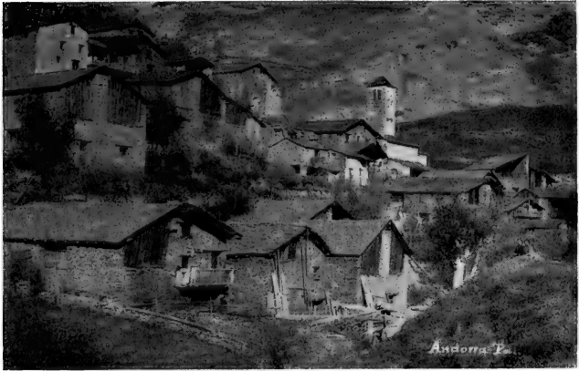
FIG. 86.—Pal, a typical village of Andorre, showing slate roofs and stone construction of houses. Note the terraces on the bare rock hillside back of the village. Every foot of soil is made available for cultivation.
