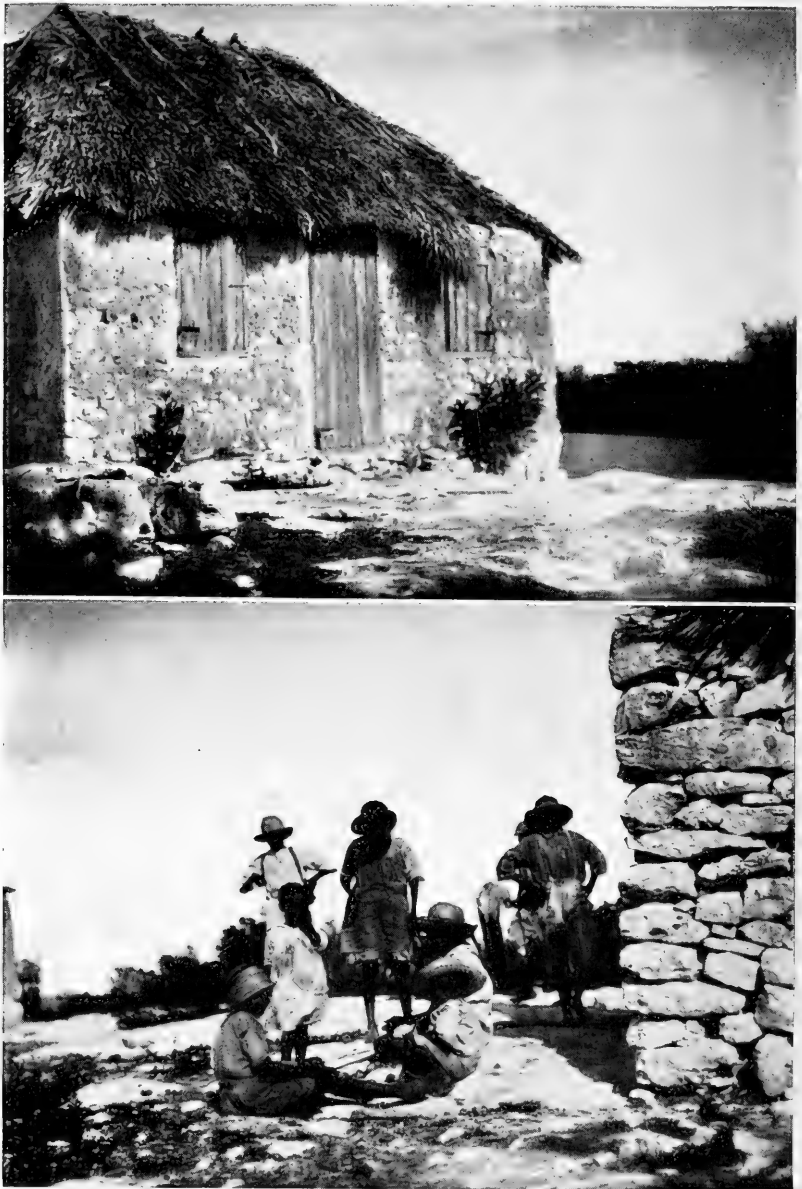
FIG. 39.—Upper: A native house of San Salvador. These are practically all built of coral limestone and usually thatched with palm. Lower: A group of native boys. The native population of San Salvador is black, practically unmixed, and of splendid physique.
