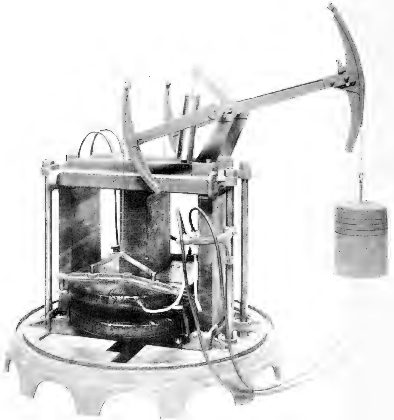
CONSTANT CURRENT TRANSFORMER, 1900.
