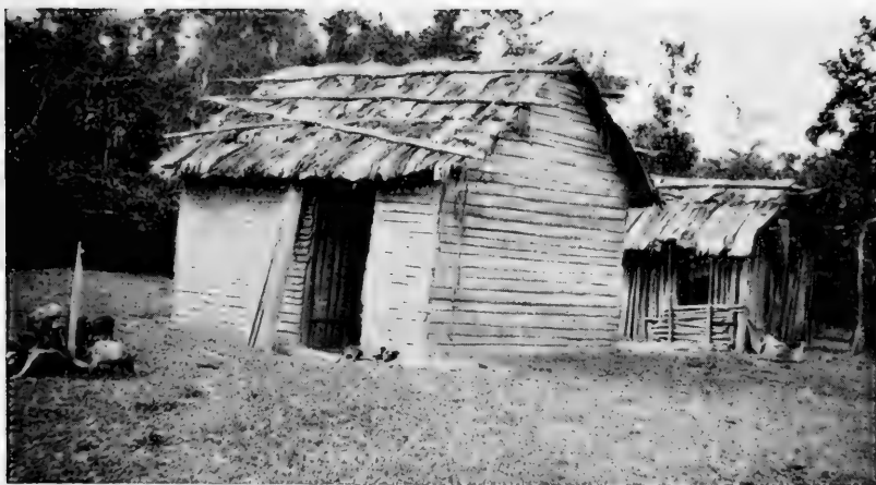
FIG. 44.—A typical house near Jovero. The roof is formed of the sheathing leaf-bases of the royal palm ( Roystonea ).
