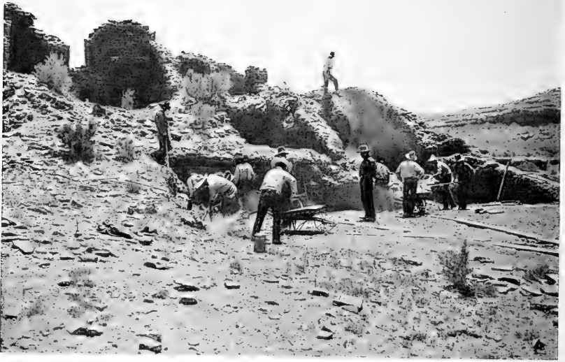
FIG. 72.—This view of work in progress on the west side of Pueblo del Arroyo illustrates the extent to which fallen masonry and blown sand will accumulate. (Photograph by O. C. Havens. Courtesy of the National Geographic Society.)
