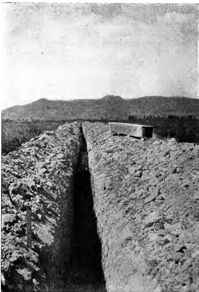
FIG. 27.— WOOD DRAINS BEING USED TO DRAIN BOGGY ALKALI LAND.
