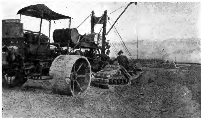
FIG. 29. — DRAINAGE MACHINE WITH THE DIGGING WHEEL IN THE TRENCH.
