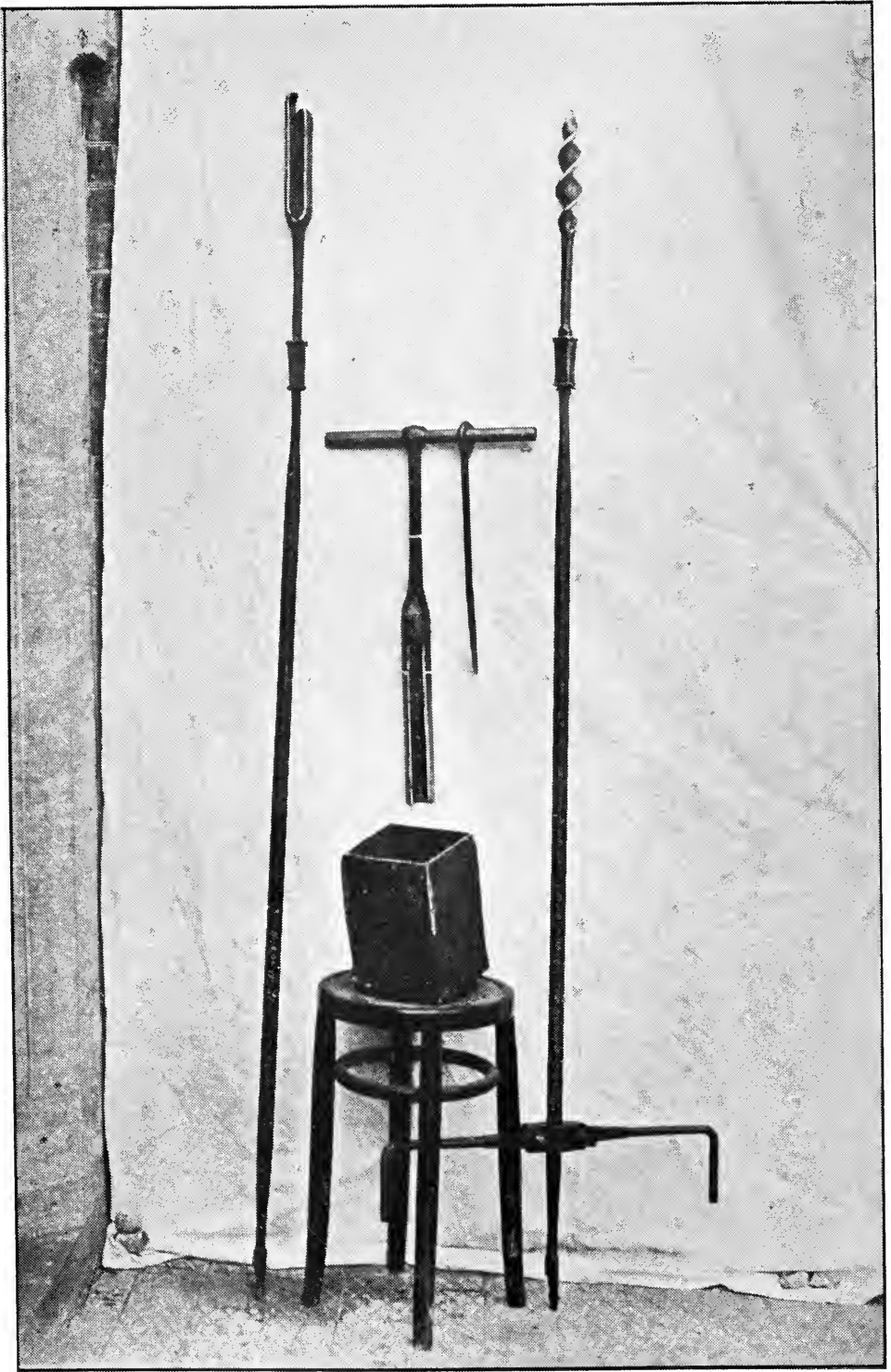
FIG. 1.—Photograph of Soil-sampling Tools.
