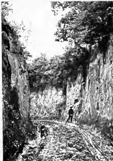
FIG. 62.—A road through a deposit of deep loess along the lower Illinois River. The deposit is 30 to 50 feet deep. The vertical walls are characteristic.
