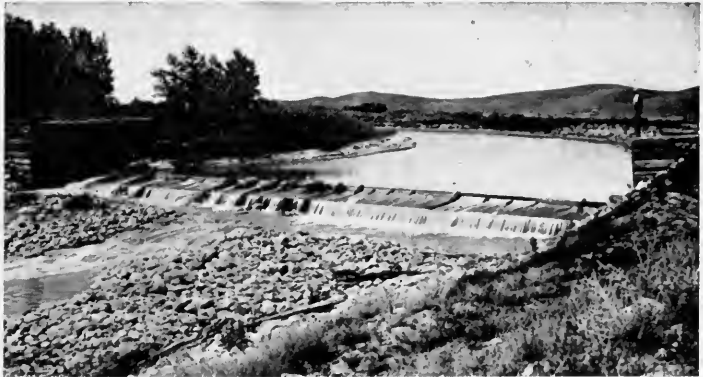
FIG. 9.—The material carried and rolled by streams gives them their great eroding power. (U. S. Reclamation Service.)
