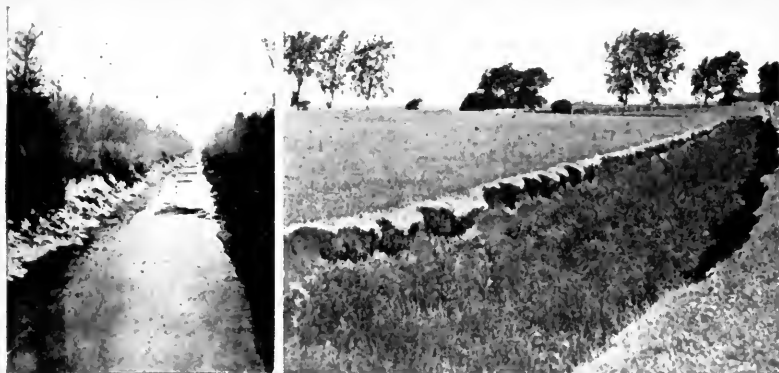
FIG. 98.—The obstructions interfere with the current and cause deflections. (H. C. Wheeler.) FIG. 99.—Ditch gradually being filled by soil due to current being retarded by grass. (C. C. Comstock.)
