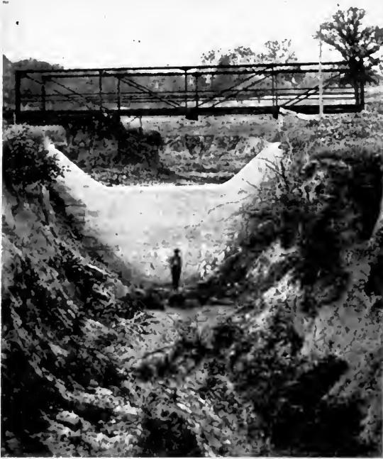
FIG. 188.—Filling a gully by means of a concrete dam.
