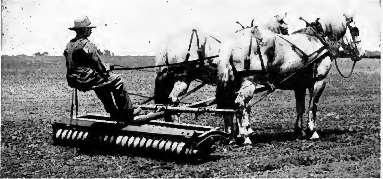
FIG. 152.—The culti-packer, a form of corrugated roller, showing the work done.
