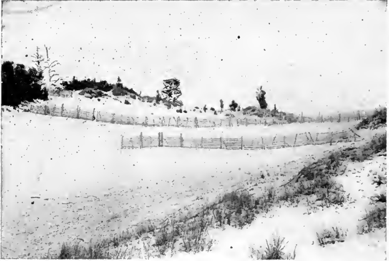
FIG. 55.—Fences being used to check the movement of sand. (U. S. Dept. of Agriculture.)
