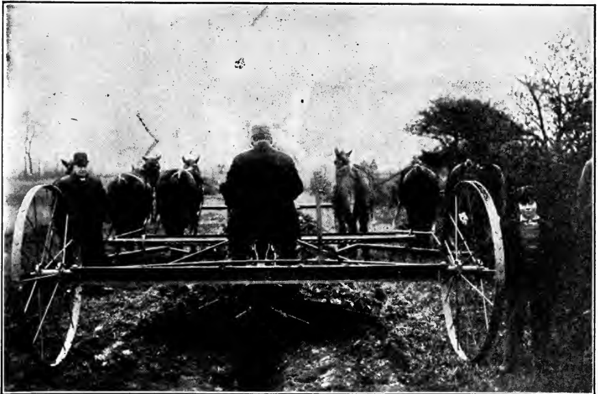
THE DITCHER IN OPERATION.
