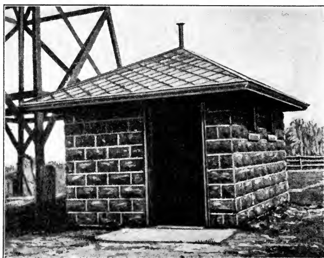
A CONCRETE BLOCK ICE HOUSE. 1
