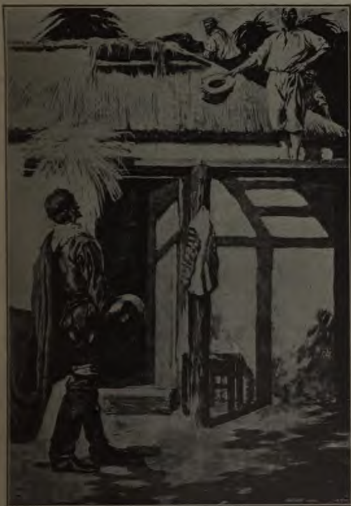
"Balboa . . . Engaged in Superintending the Roofing of a House "
