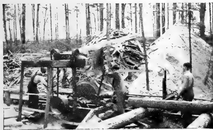
FIGURE 46.—Slabs and edgings can provide raw material for the pulp mill, where transportation is practicable.
