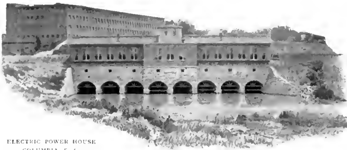
ELECTRIC POWER HOUSE COLUMBIA, S. C.
