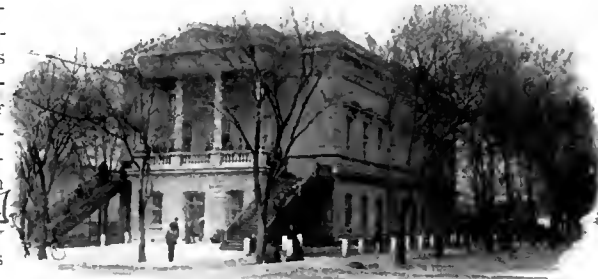
COUNTY COURT HOUSE, COLUMBIA, S. C.
