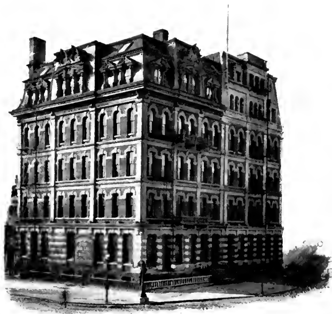
THE SOUTHERN RAILWAY BUILDING, WASHINGTON, D. C.
