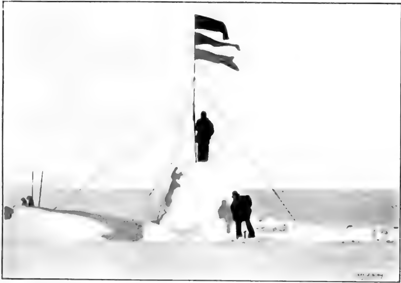
BUILDING THE BULL DEPOT.
