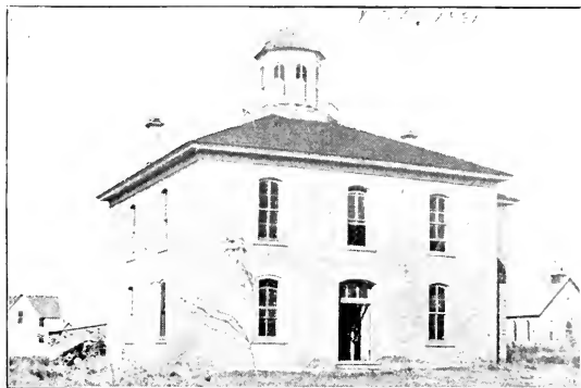
BUILDING THE COURT HOUSE.
