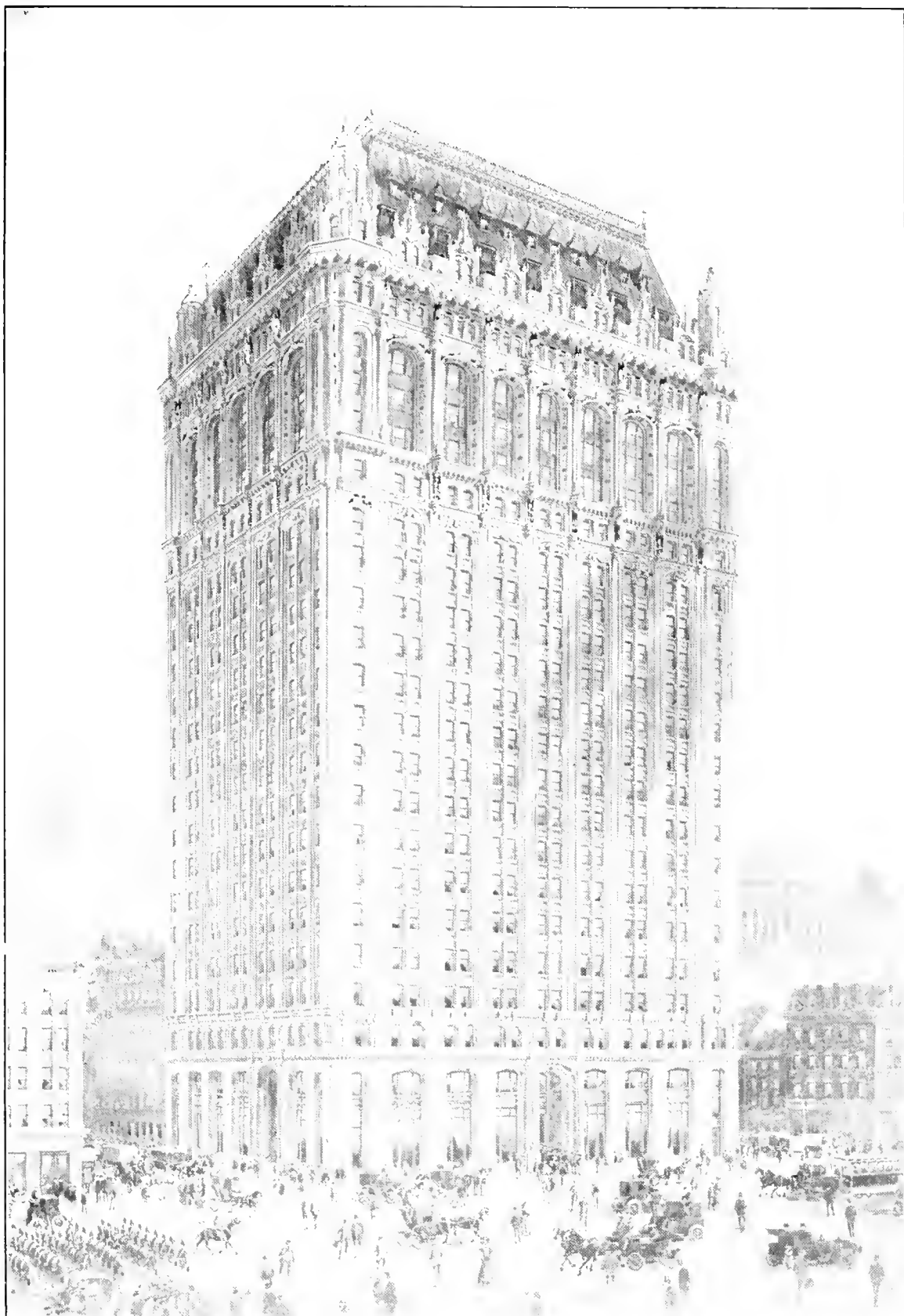
West Street Building
