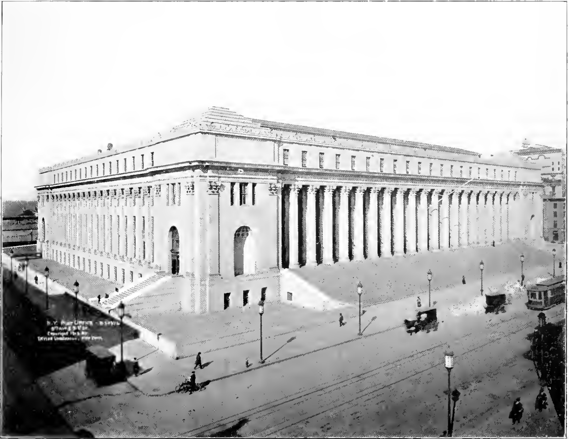
New Post Office, Eighth Avenue and Thirty-first Street
