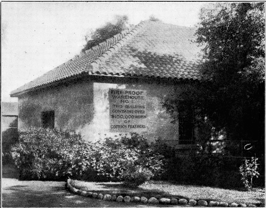
A Fire Proof Warehouse at the Cawston Farm, South Pasadena
