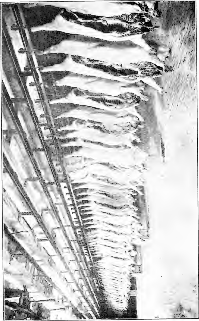
KINGAN'S KILLING DEPARTMENT. HOG-HANGING ROOM FOR 3,000 HOGS.
