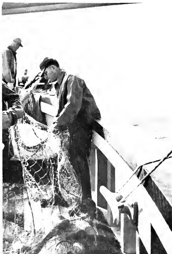
Figure 6.--After coming around the sheave on the anchor winch (to the left of the photo) the gill nets were cleared on their way to the stern of the John N. Cobb .
