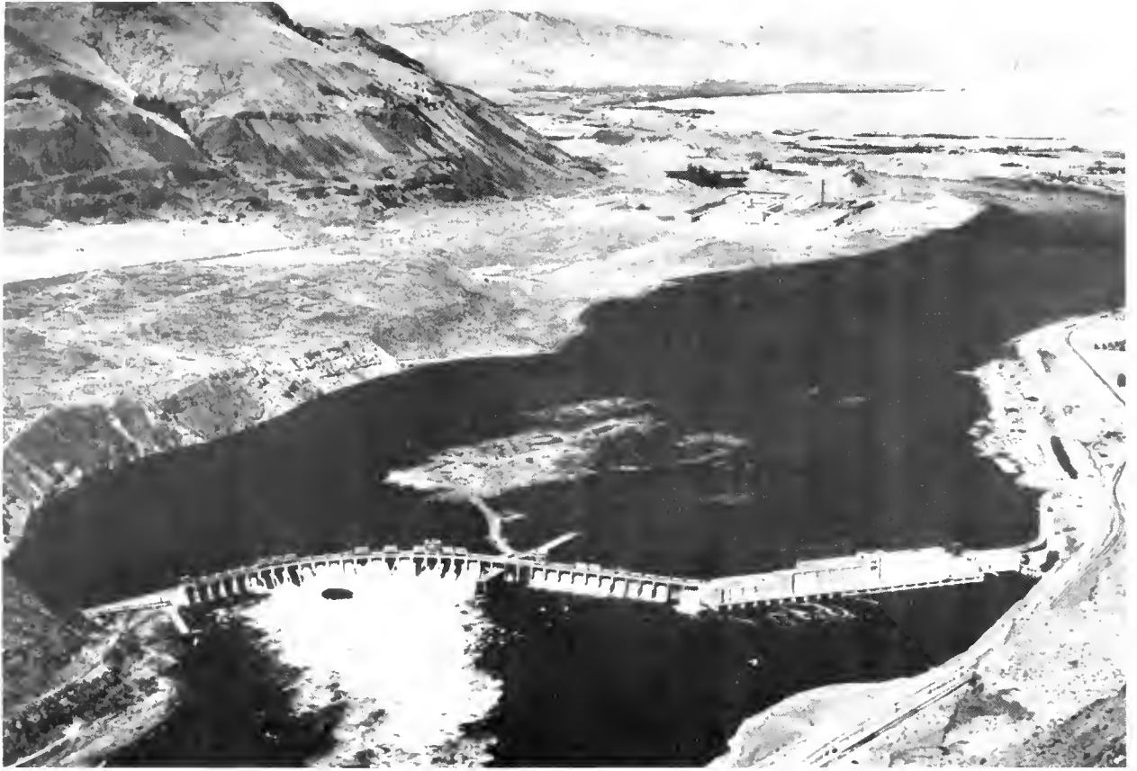
Rock Island Dam, Columbia River, Wash.
