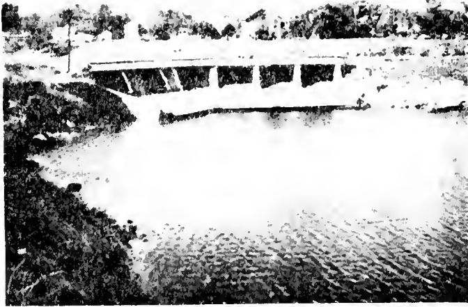
Figure 8.--Power dam in Cheboygan River at Cheboygan, Michigan.
