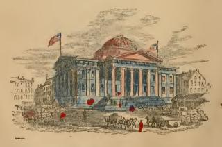
built on three thousand piles; on the top of these is a granite platform, and on that the foundation of the walls was laid."
