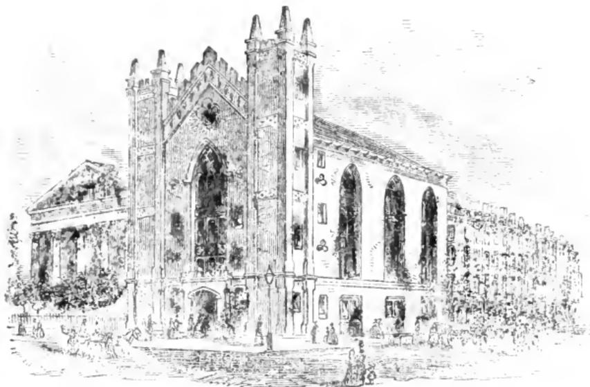
nies, in 1630. It is built of granite, with towers sixteen feet square, surmounted with battlements and pinnacles. The doors and windows are of fine hammered granite. The blocks of granite are triangular, and it is a very handsome building. There is no other in Massachusetts like it.
