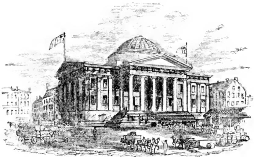
built on three thousand piles ; on the top of these is a granite platform, and on that the foundation of the walls was laid.”
