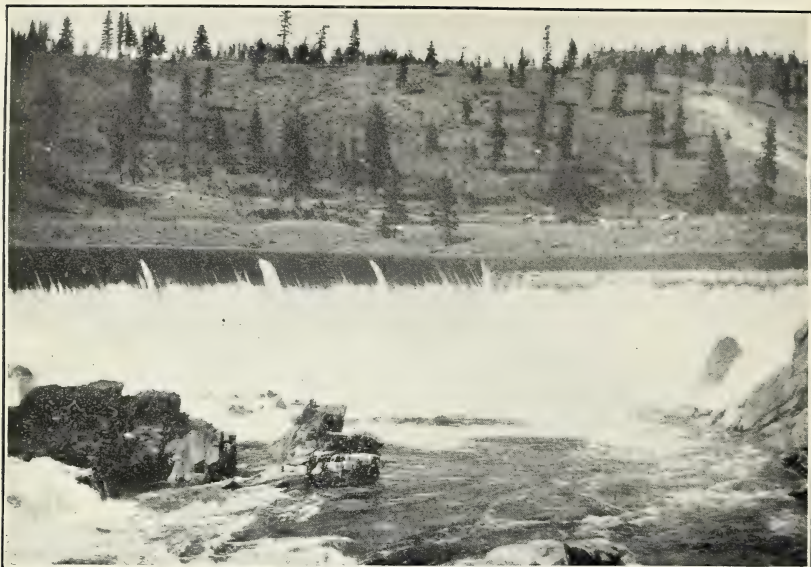
FIG. 1.—DIVERSION DAM, WASHINGTON POWER CO., NEAR SPOKANE, WASH. Built at the Little Falls plant in the form of an "L" to gain crest length
