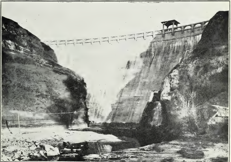
FIG. 2.—EAST PARK DAM, ORLAND PROJECT, CALIFORNIA.
