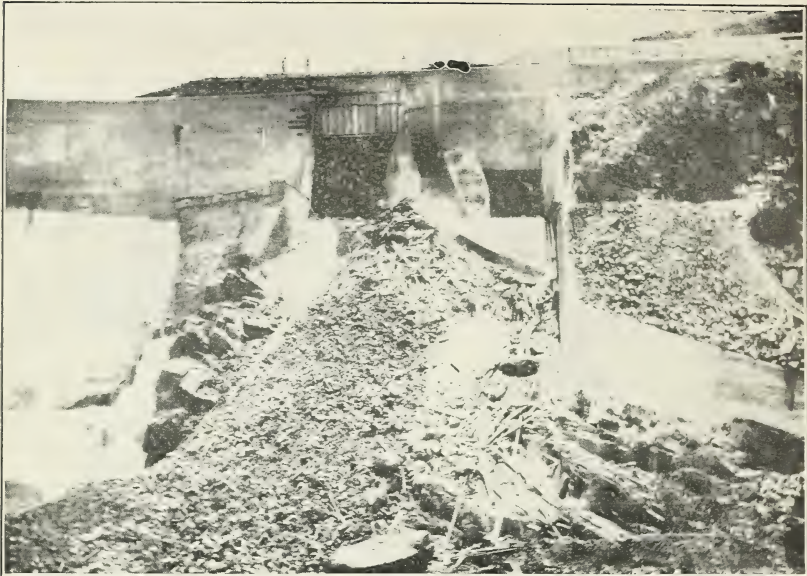
FIG. 1.—OUTLET OPENING FOR OVERPOUR SPILLWAY AT SOUTH END OF SWEETWATER DAM, CALIFORNIA.
