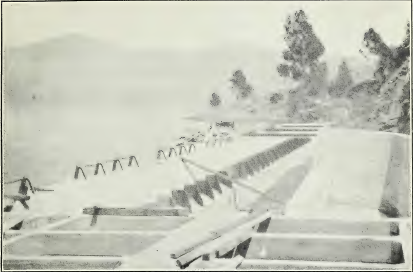
FIG. 1.—SOUTH OVERFLOW SPILLWAY, SWEETWATER DAM, CALIFORNIA. Showing inclined braces along top of spillway crest to support flashboards.
