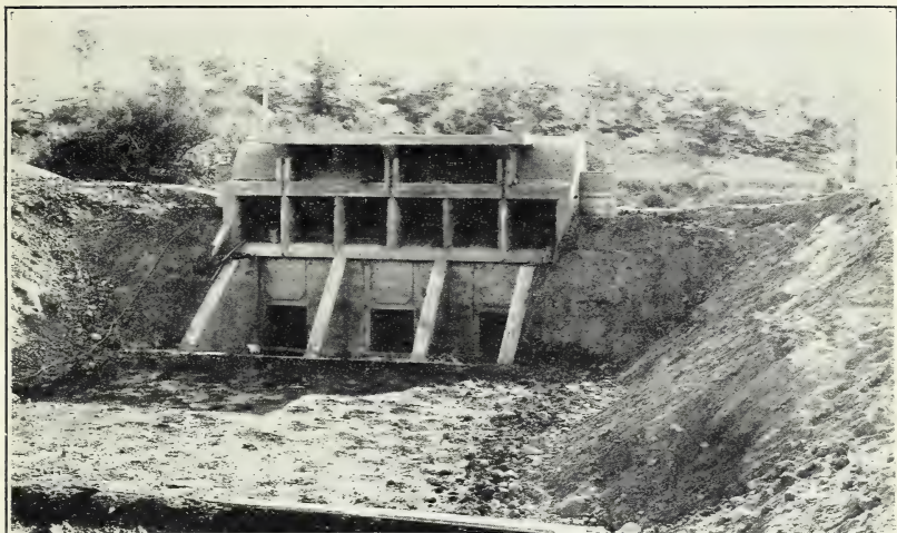
FIG. 1.—INTAKE END OF SIPHON WASTEWAY ON MAIN CANAL OF SUN RIVER PROJECT.
