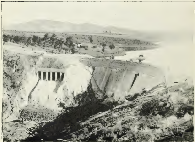
FIG. 2.—SWEETWATER DAM AS COMPLETED AFTER THE FLOOD OF 1915.
