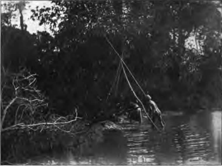
FIG. 9. —A “wala” at Hanwella being baled out by means of an irrigation scoop (“yotu-kanda”) over a low bund.
