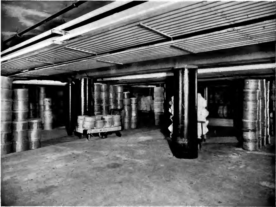
COLD STORAGE WAREHOUSE
