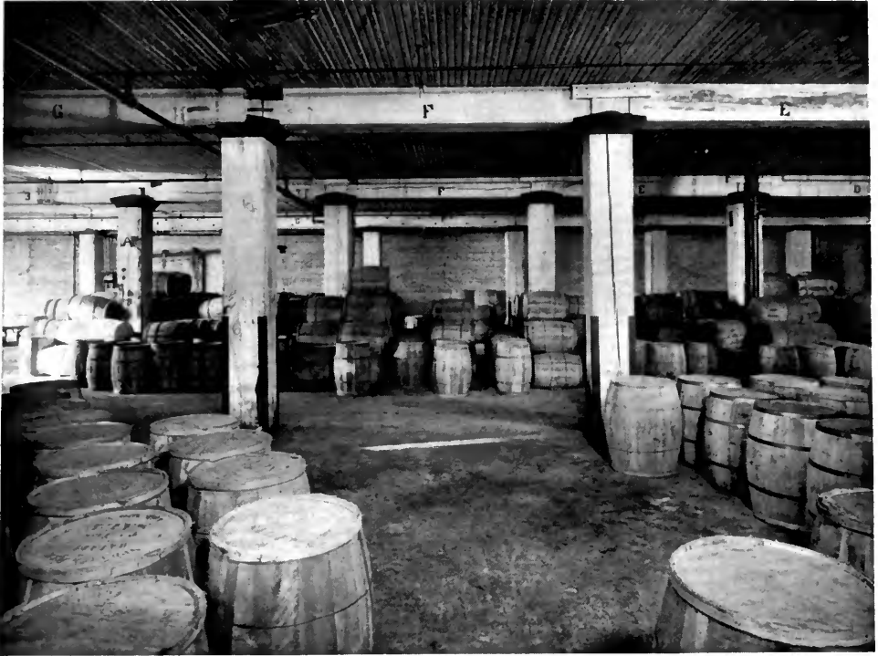
SUGAR AND SALT WAREHOUSE
