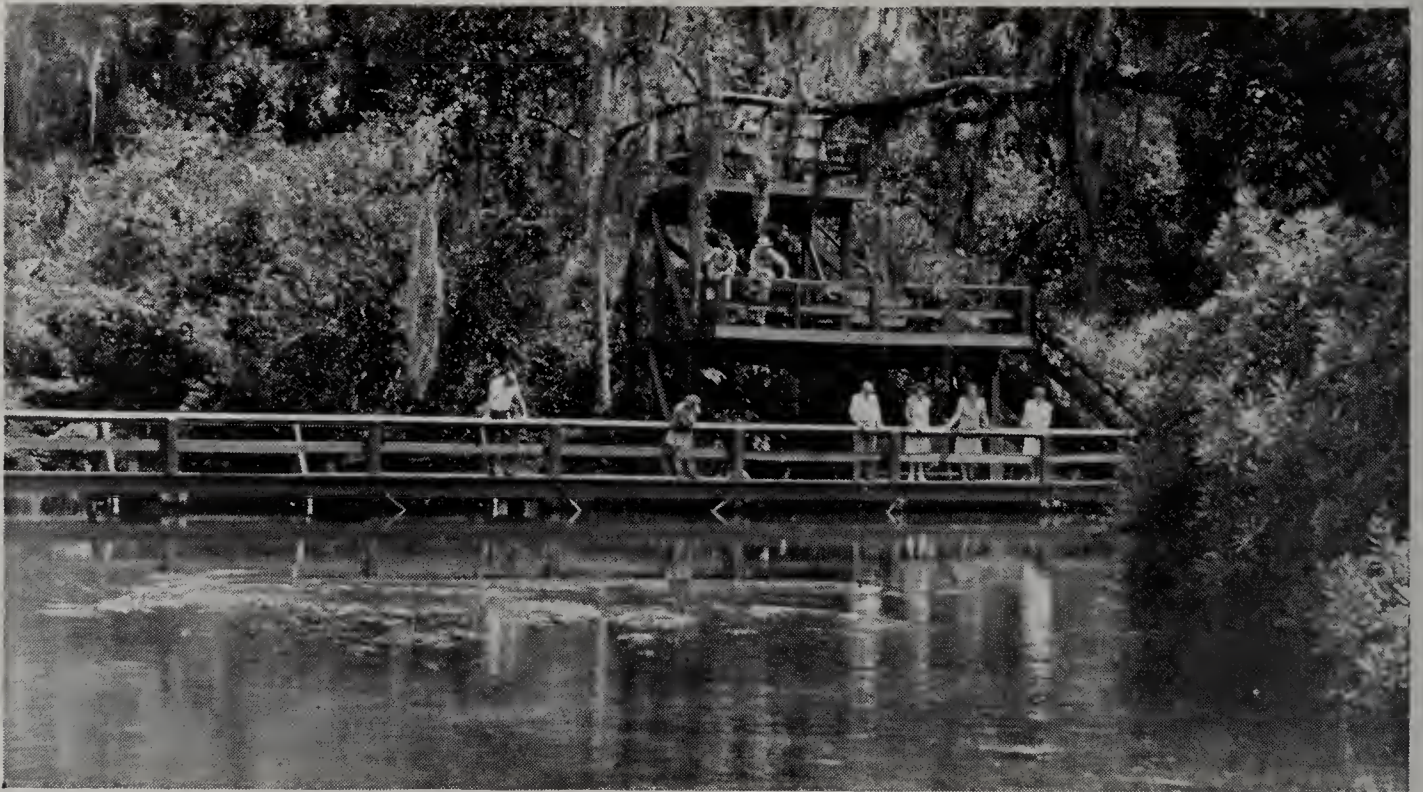
FIGURE 9. View of the headpool of Homosassa Springs , showing platforms from which the underwater scenery can be seen.
