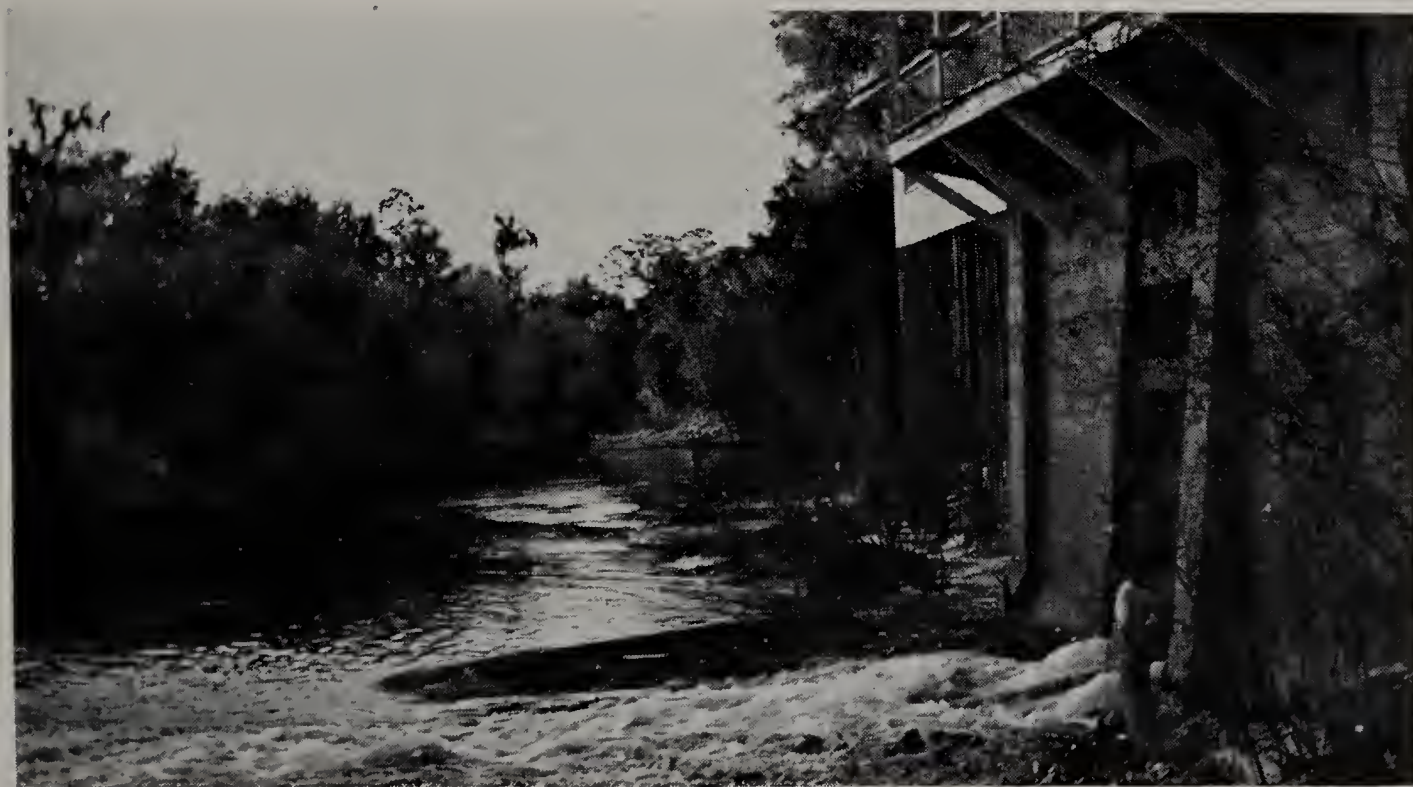
FIGURE 13. View of discharge vent at White Springs , which is located inside the building shown to the right of the picture.
