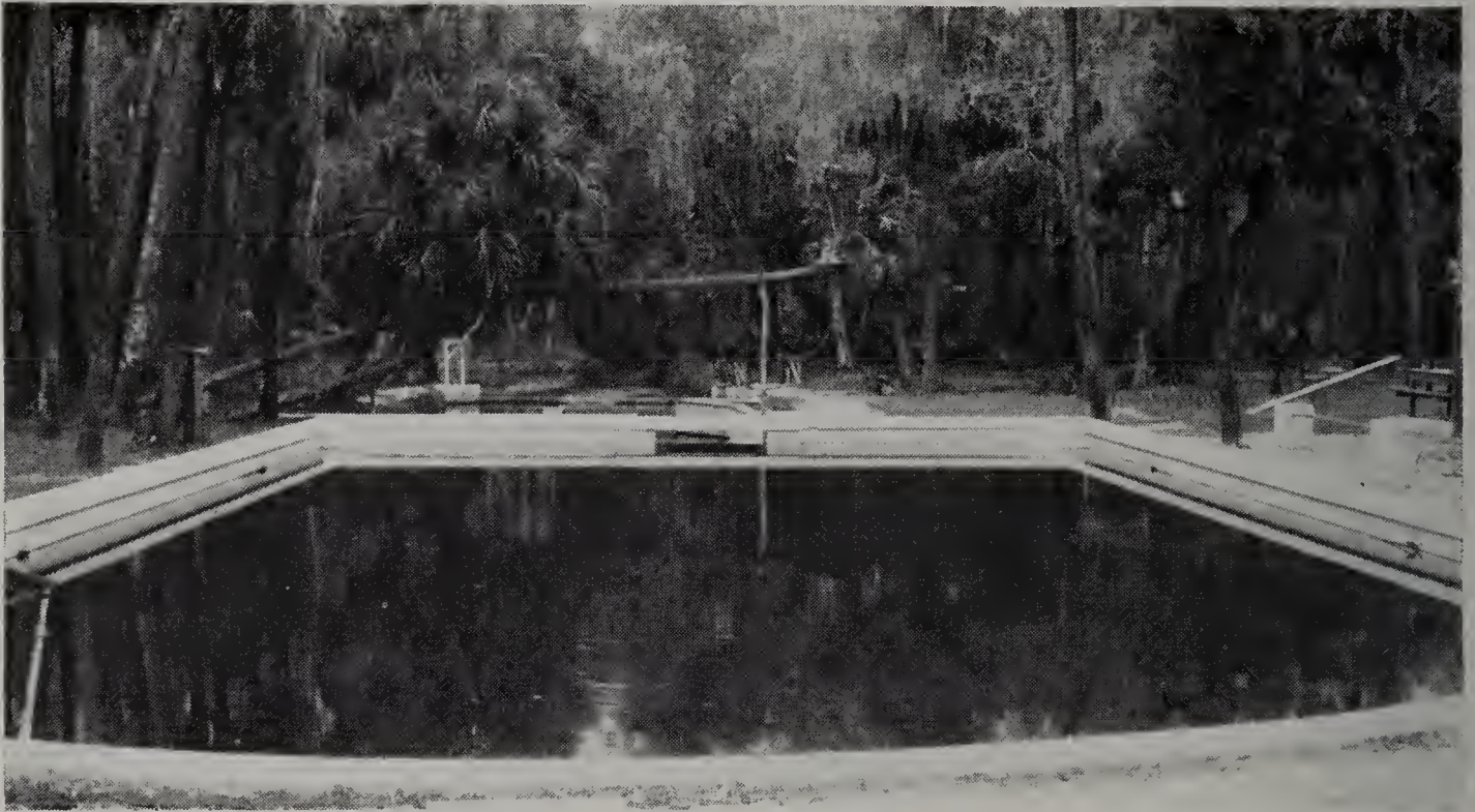
FIGURE 30. Pool basin at Palm Springs , Seminole County. Photograph taken 1935.
