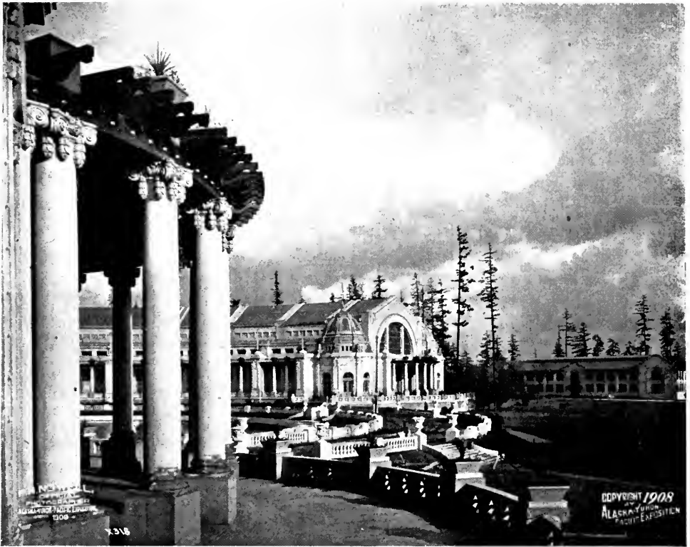
FROM THE STEPS OF THE AGRICULTURE BUILDING, NOVEMBER, 1908.
