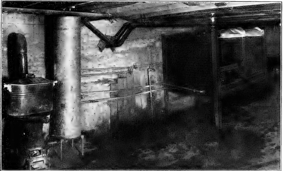
WASH ROOM AT MORRIS FARM, LEBANON, OHIO
