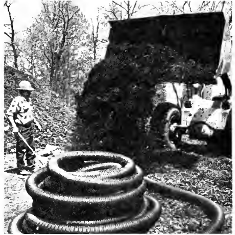
Fig. 3. A 20' x 60' bed of wood chips is laid down for good distribution of air.
