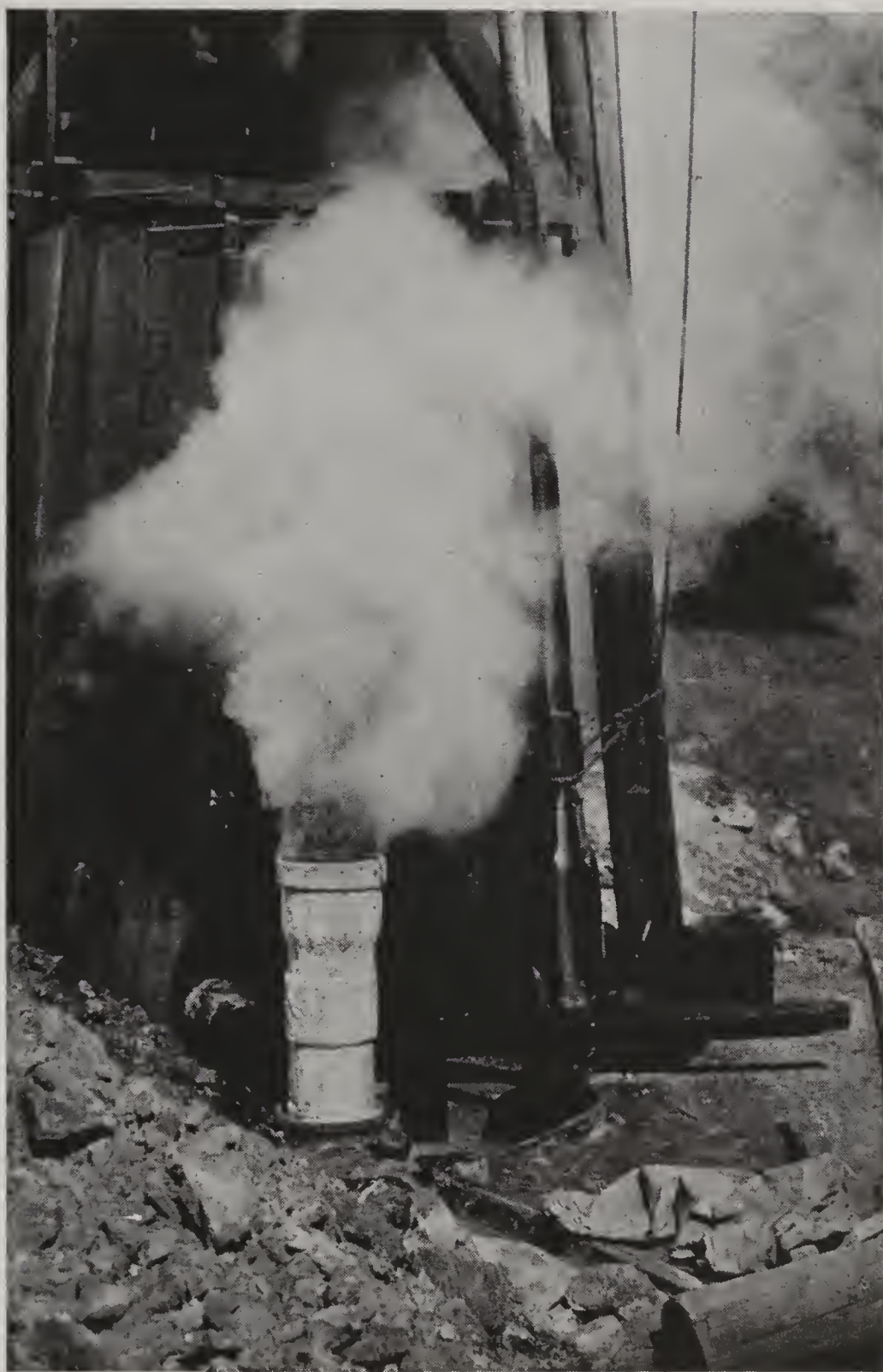
Fig. 30—Well No. 3 as it appeared in 1925. Casing is coated with opal formed by evaporation of small amount of water constantly thrown out with steam.
