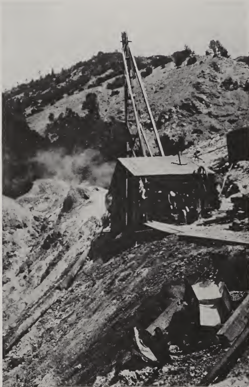
FIG. 19—Drilling first well. The Geysers, 1922.
