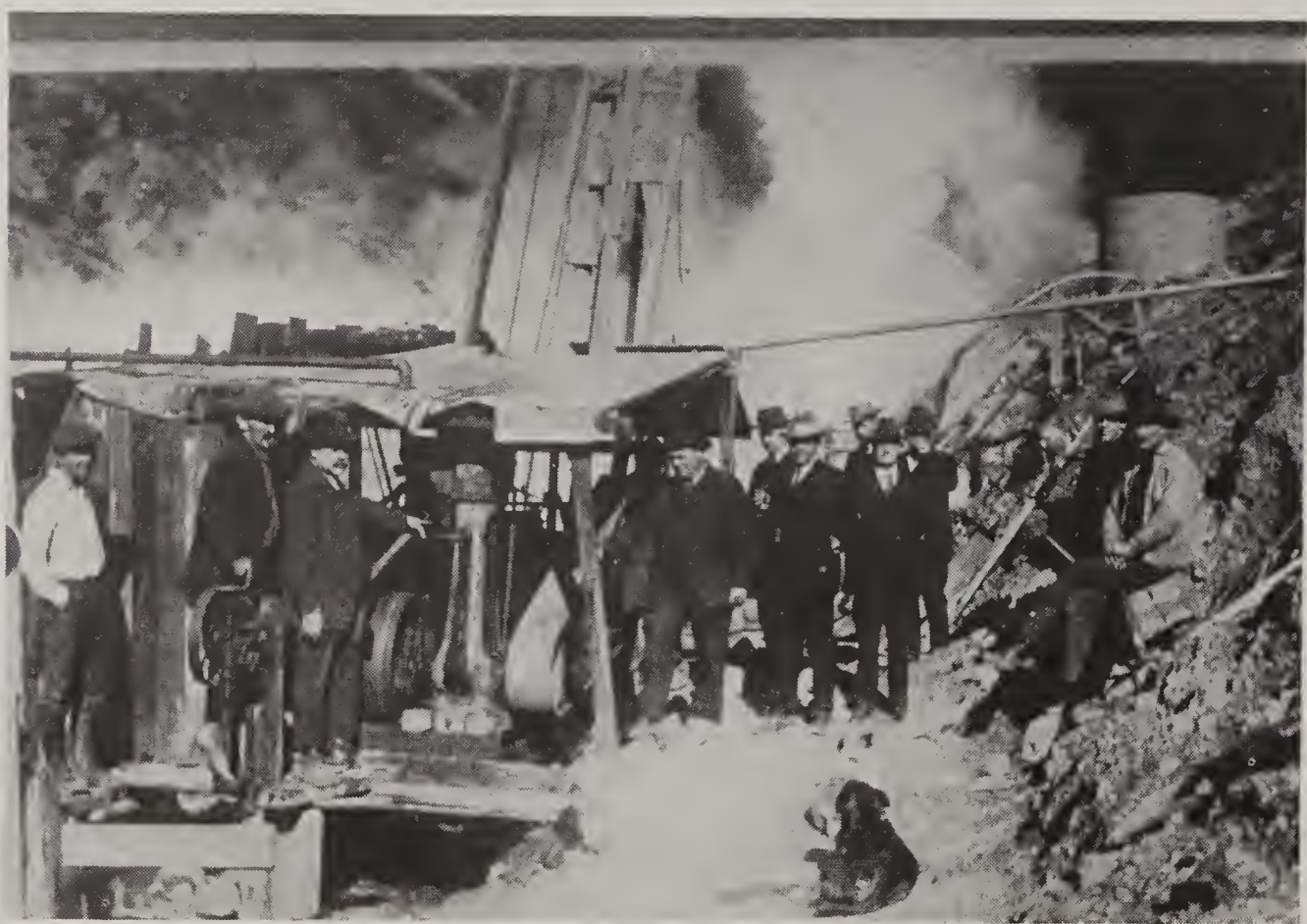
FIG. 21—Drilling second well with steam power from first. Photo obtained from J. D. Grant.
