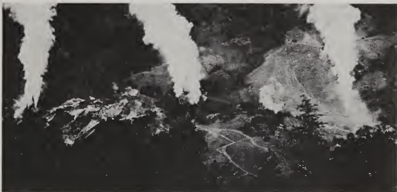
FIG. 23—Wells open. No. 1 and No. 2 left, No. 4 center, No. 5 right and No. 6 partially closed down between No. 4 and No. 5. 1925.
