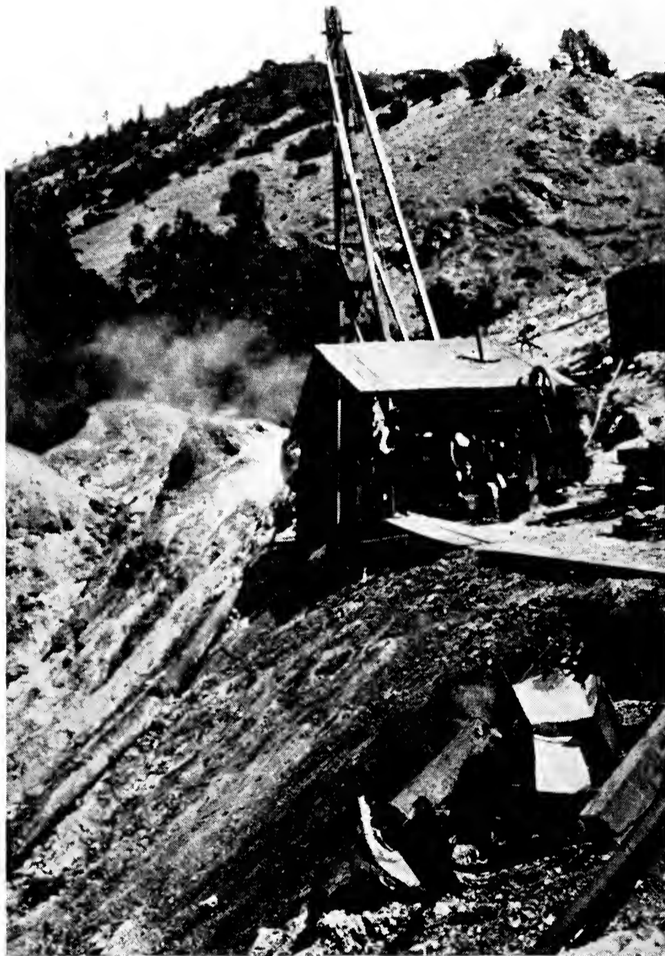
FIG. 19—Drilling first well. The Geysers, 1922.
